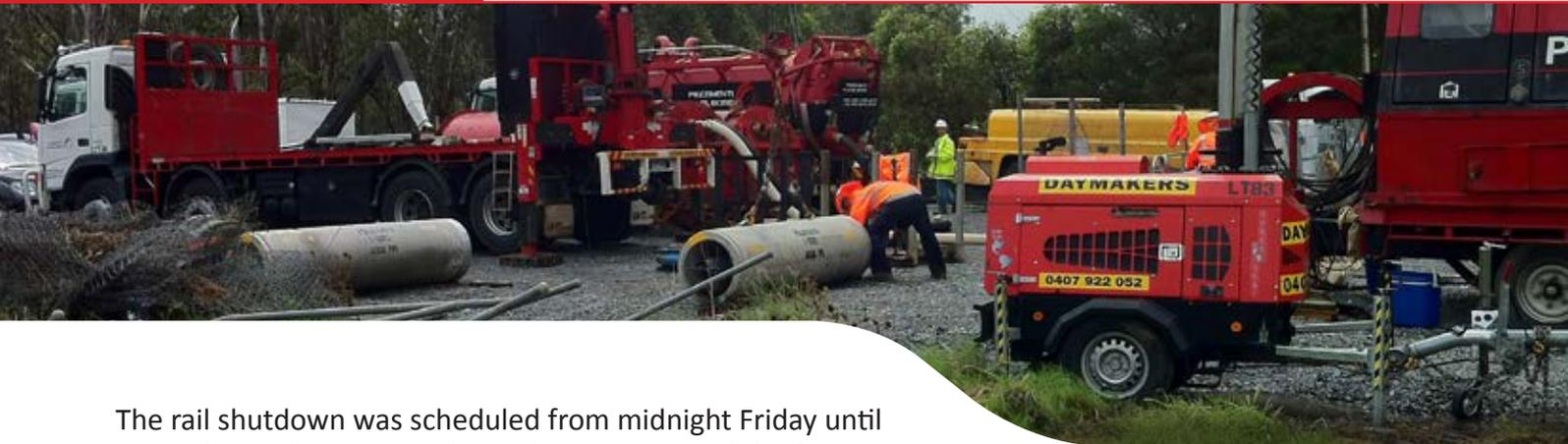
The rail shutdown was scheduled from midnight Friday until midnight Sunday. It was planned to microtunnel the first 16m prior to the shutdown. The remaining 43 m would be microtunnelled (with 2 crews working consecutive 12 hour shifts) and the annular space between the pipes and the microtunnel grouted during the shutdown.
