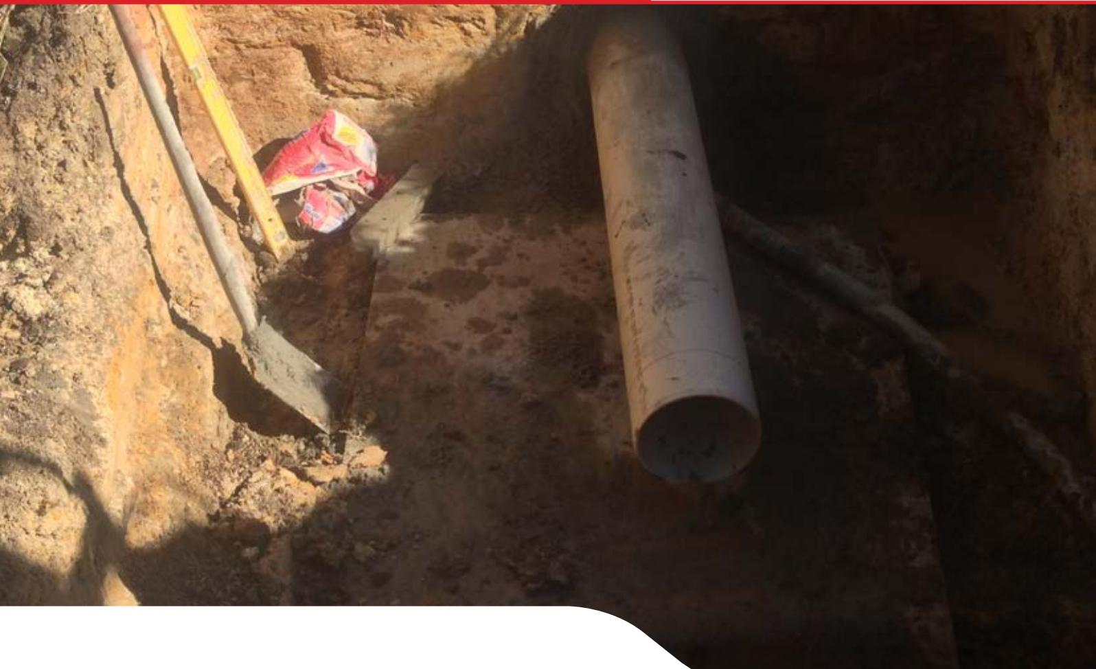
The connection to the existing sewer system for an exclusive residential development at Little Bay, required a steeply graded line to be drilled under an existing golf course.
