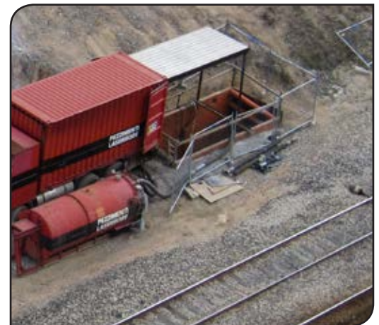
+ Proximity of shaft to Railway Line
