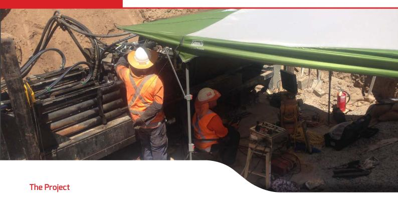
For this diameter Pezzimenti has developed an auger extraction system which is used to transport the material from the face back to the shaft. Augers use less water than vacuum extraction which is used for smaller diameters.
