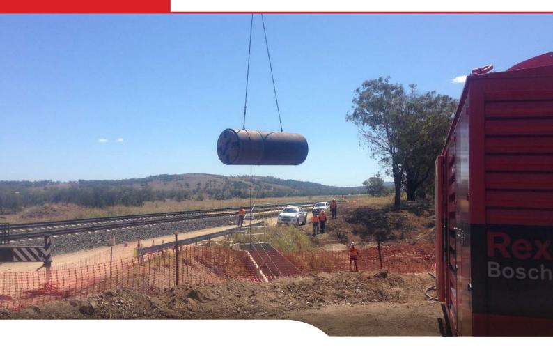
The Upper Hunter Valley Alliance was formed between Leighton Contractors and ARTC in 2009 to deliver a significant program of civil and track works on the Hunter Valley rail network between Singleton and Werris Creek. As part of these works a new Ø1050 stormwater culvert was required to be installed under the rail line near the town of Willow Tree.
