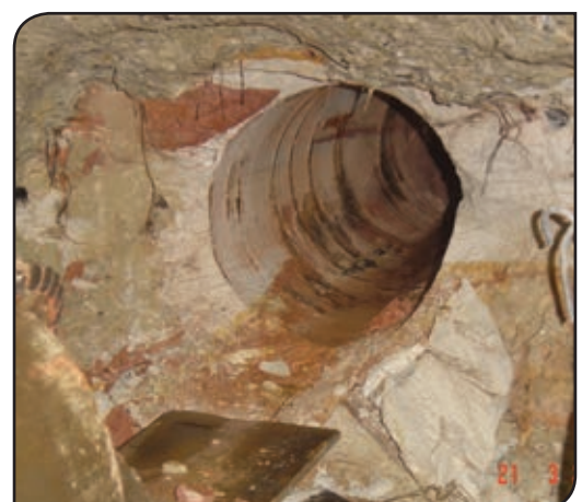
+ The 2nd tunnel.
