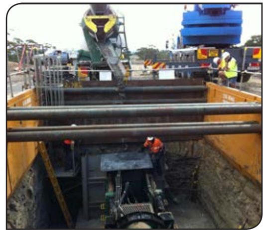
+ Jacking Frame secured in Shaft
